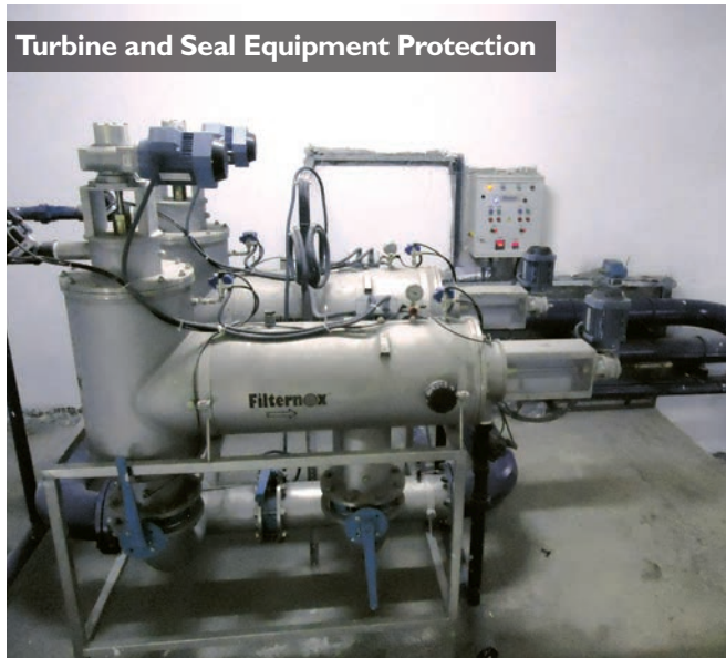
Turbine and Seal Equipment Protection
