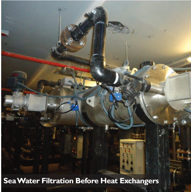
Two Stage Filtration of Sea Water Before RO and Desalination
