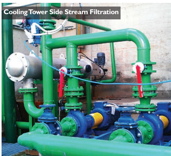
Cooling Tower Side Stream Filtration
