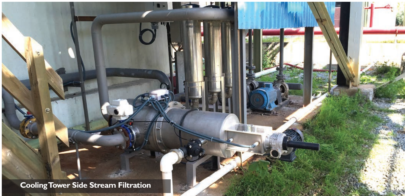
Cooling Tower Side Stream Filtration
