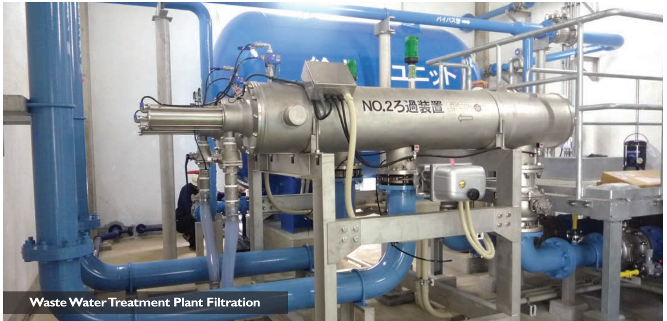
Treated Waste Water Filter Station
