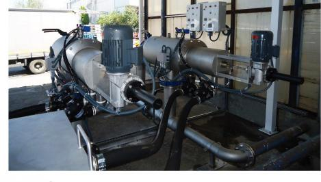
Filternox® SPT-WBV-MR model filtration system has a patented design that enables effective filtration of water containing coarse and fine particles. SPT-WBV-MR, which has a double-effect cleaning system with brush and vacuum nozzle, is automatically cleaned from coarse particles on the surface of the screen by brush and then fine particles from the surface of the screen by vacuum nozzle. cleaning.
