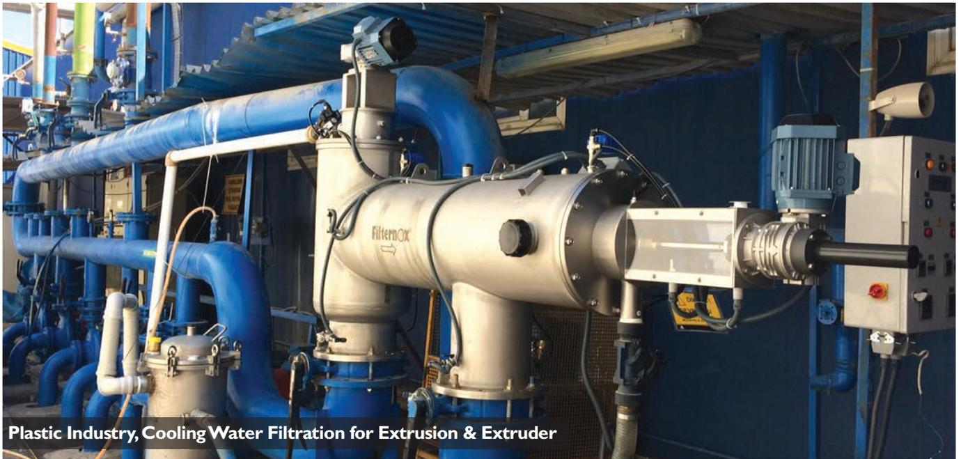
Plastic Industry, Cooling Water Filtration for Extrusion & Extruder
