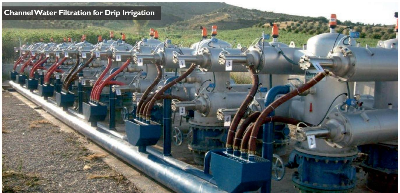
**Channel Water Filtration for Drip Irrigation**
