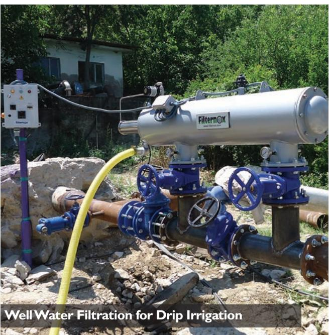
**Well Water Filtration for Drip Irrigation**
